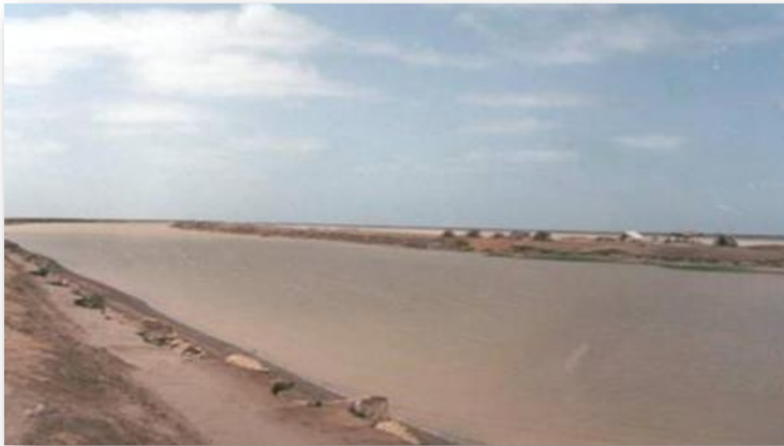
Tidal link drain Before Cyclone 2A 1999
